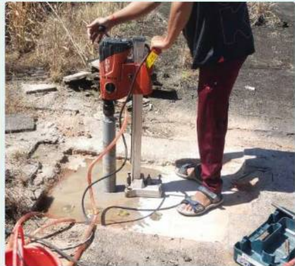
Extraction of concrete core specimen from Roof Slab
