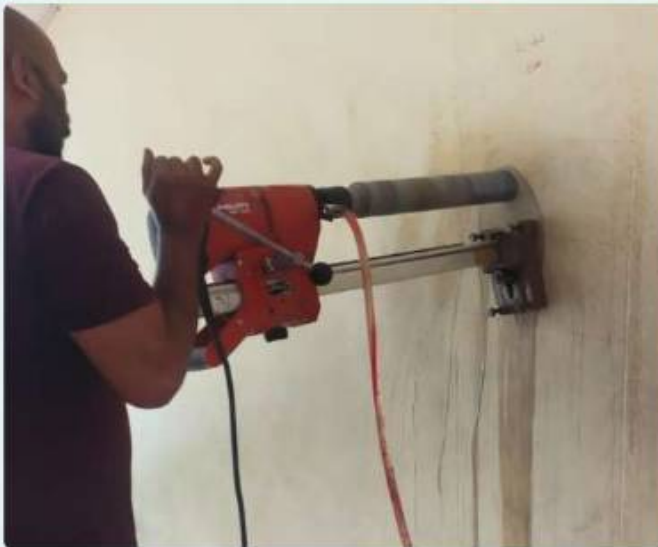
Extraction of concrete core specimen from Roof Slab
