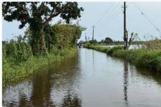
Waterlogged Pullu-Manakkodi road
