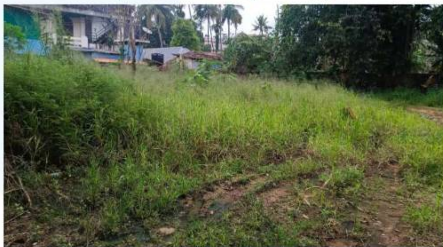
Sand compaction pile for foundation of Changanassery police station, Kottayam
