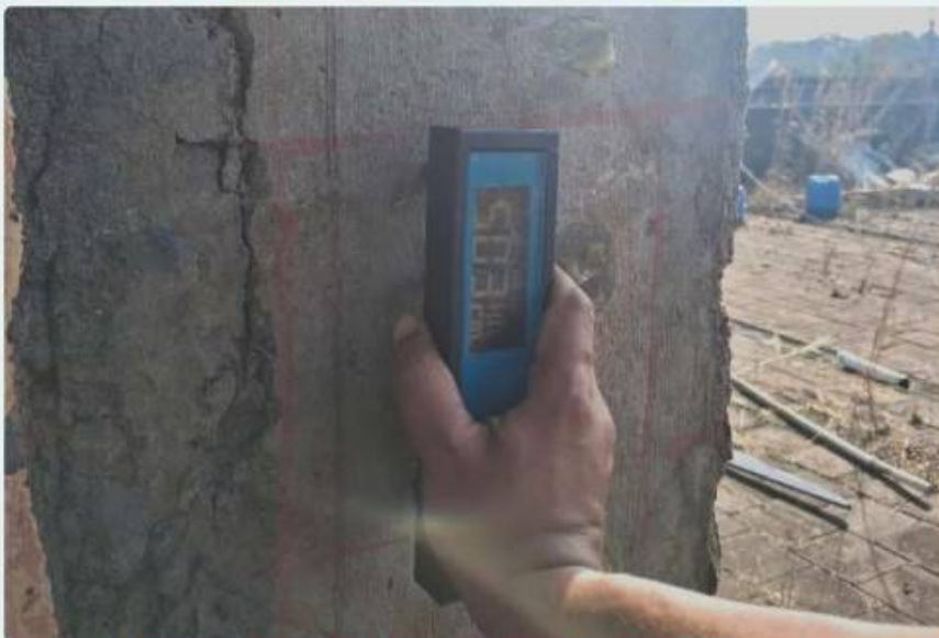
Surface Resistivity Test at Stair Column
