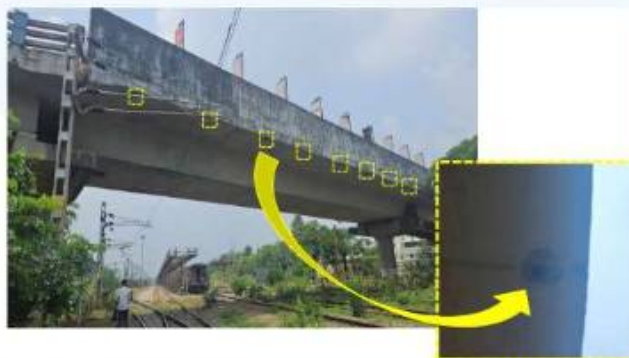
Location of drainage outlets in the RoB portion constructed by Indian Railway
