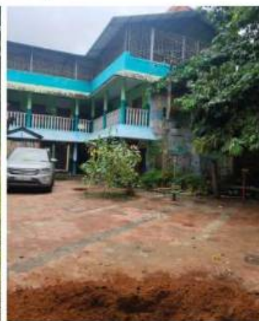
Sand compaction pile for foundation of Konchiravila UPS
