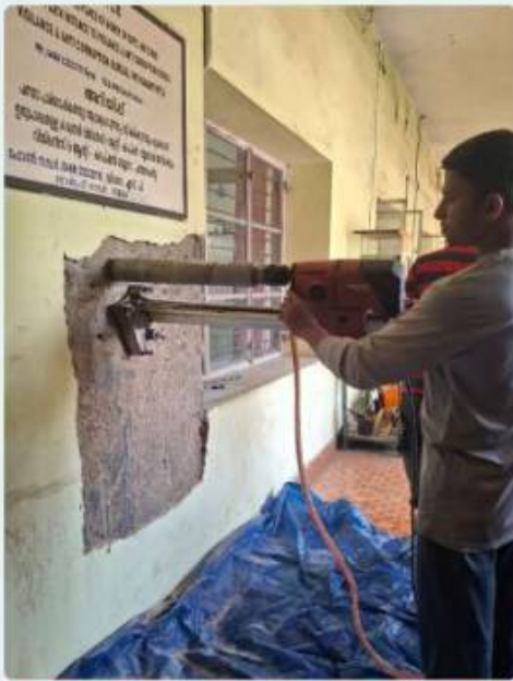
Extraction of concrete core specimen from RCC Wall
