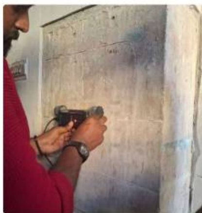
Locating rebars using cover meter
