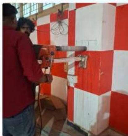
Extraction of concrete core specimen from column
